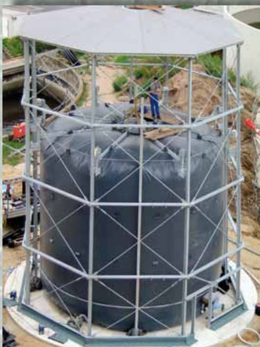
Gas holder (during installation)
