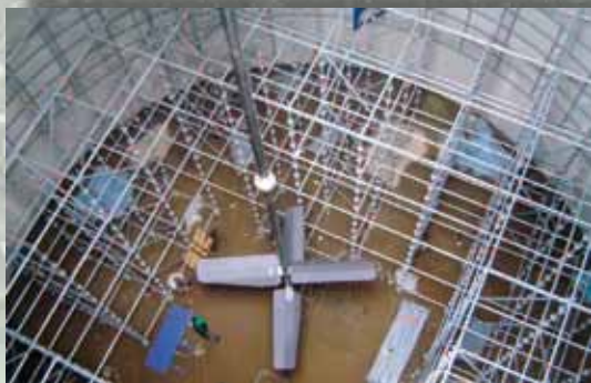
Paddle mixer in fermentation container (during installation)
